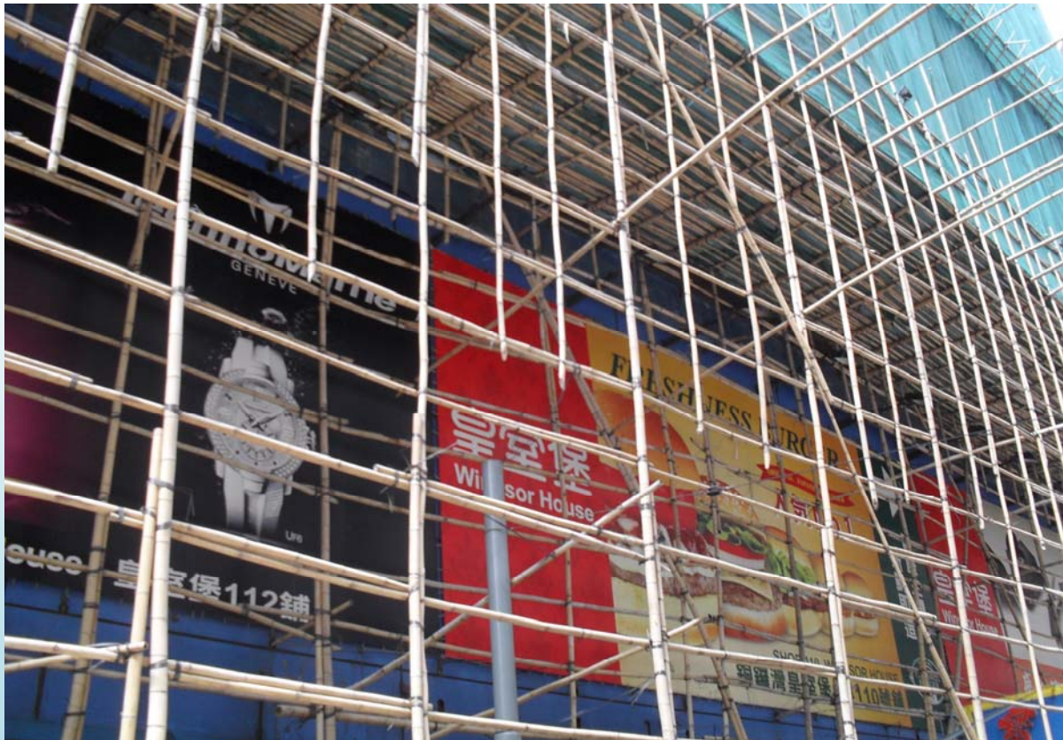
Bamboo scaffolding is a common construction material in China.
